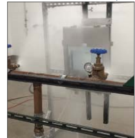
Water Ingress Testing
